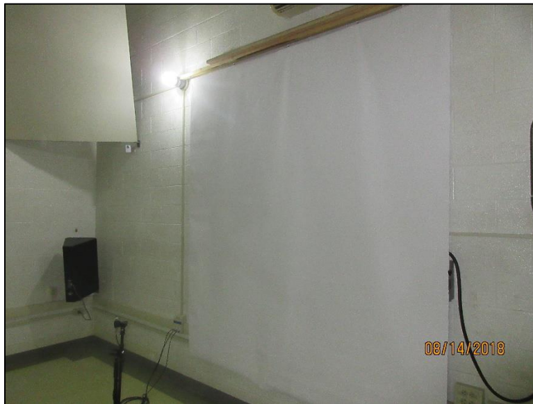
Photo No. 1 View of Installed specimen
