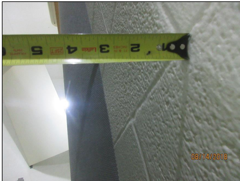
Photo No. 2 Side view of Installed Specimen
