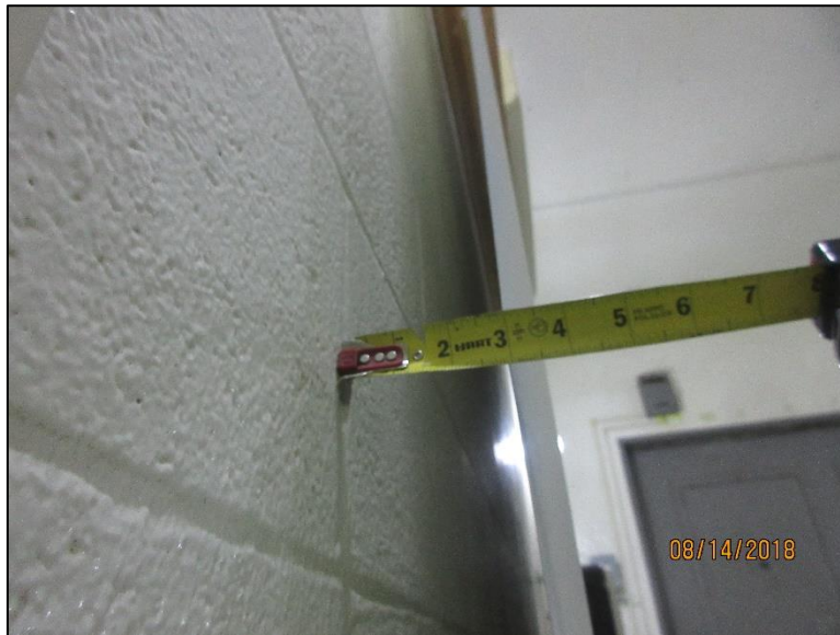
Photo No. 2 Side View of Installed Specimen
